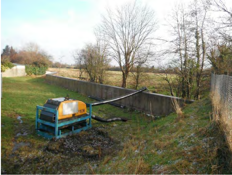
Figure 4 Photo of Derrymullen Flood Defence Wall with Surface Water Pump
